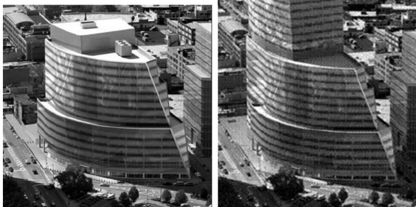
Notes: Phase I (left) and Phase II (right) Sources: Kohn Pedersen Fox (2005); Pearson and Wittels (2008)
