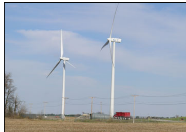
Bowling Green, Ohio Wind Farm
